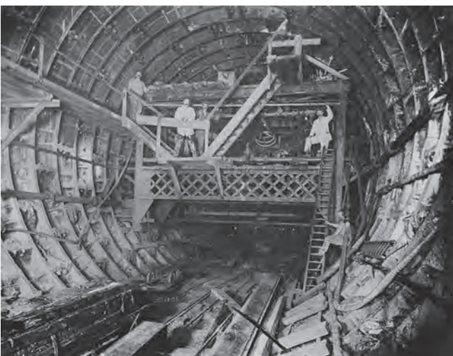
Rotherhithe Tunnel under construction (1906)
